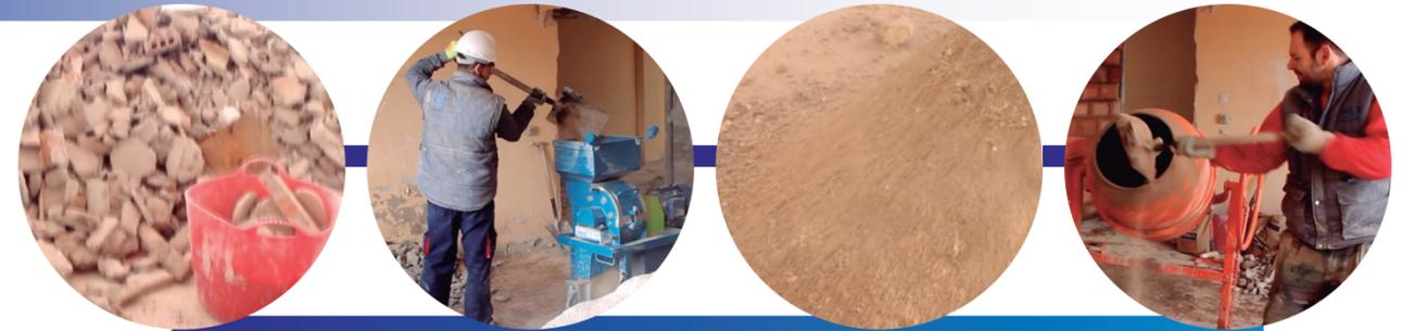
The debris processed by the TRITON is transformed in sand, that can be reuse to produce mortar/concrete.
