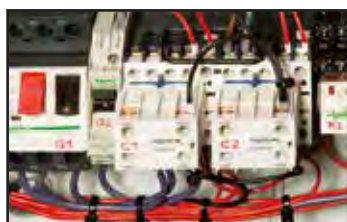
Overload magneto-thermal protection switch.
