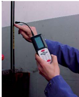
TENSION CONTROL BY VIBRATION METHOD
